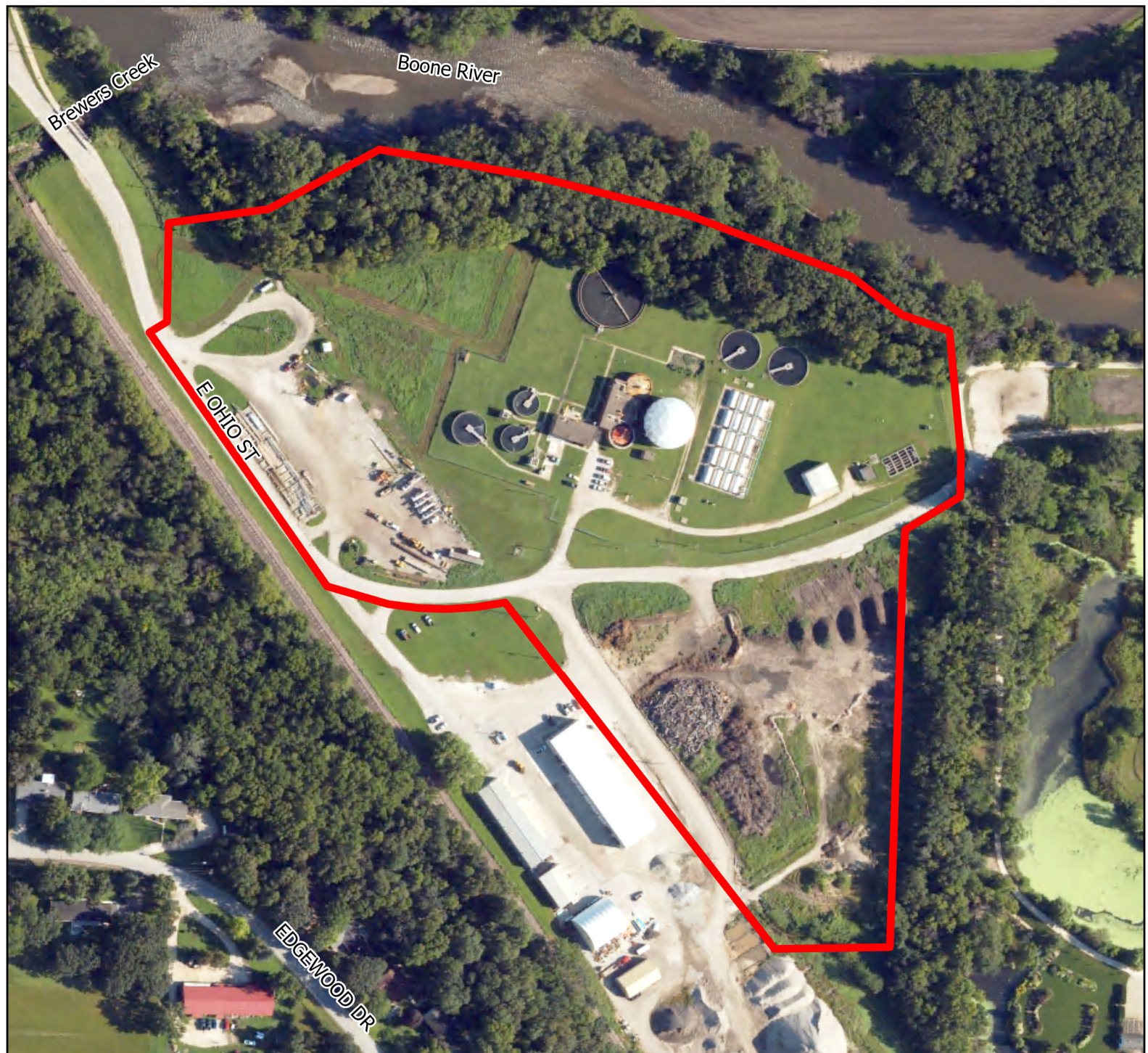
City of Webster City WWTF Improvements Webster City, IA (Hamilton County)
