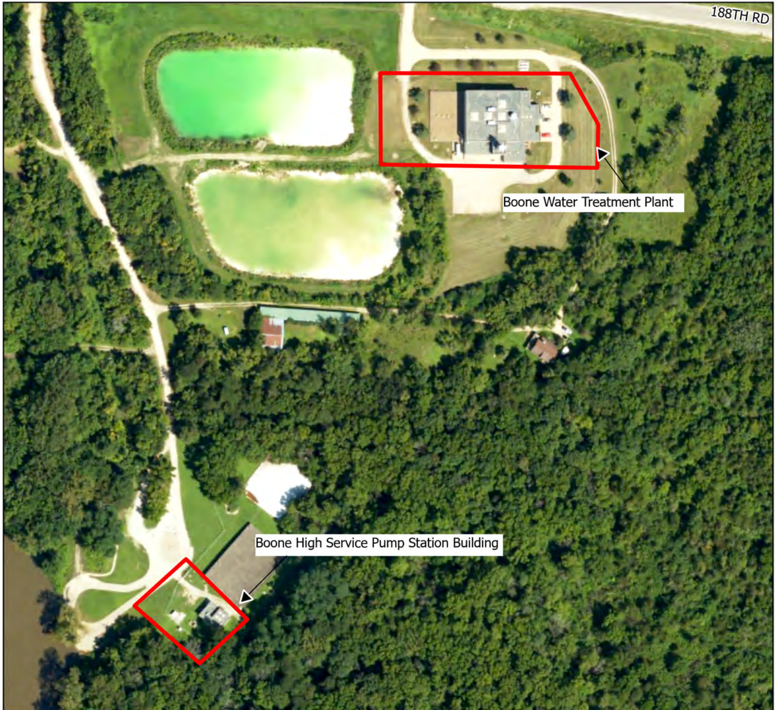
City of Boone Water System Expansion Project #2-4: High Service Pump Station Improvements Boone, IA (Boone County)
