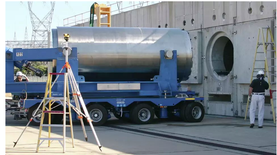
Photo: Horizontal cask loading operations Source: Dominion Energy
