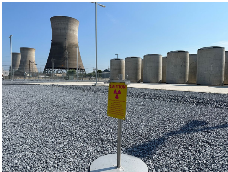
Photo: Vertical casks with cooling towers in background Source: Miriam Juckett/PNNL
