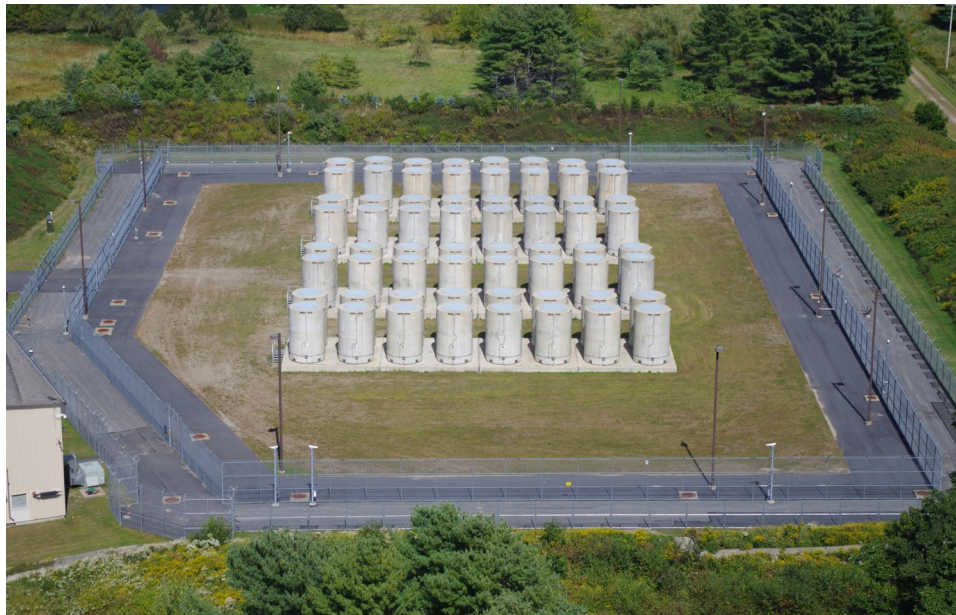
Photo: Independent spent fuel storage installation at decommissioned nuclear reactor site Source: Maine Yankee (Three Yankees)
