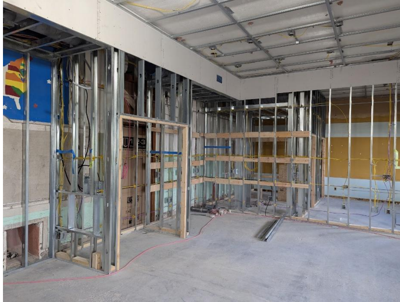
Photo 1 (Dated 9/19/25): 3rd Floor - Demo & framing complete, MEP rough-in nearly complete, drywall underway
