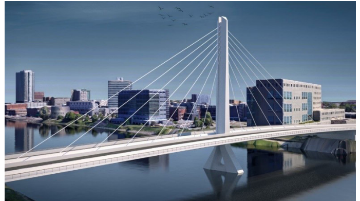
Figure 5: 8th Avenue Cable Stay Bridge Concept
