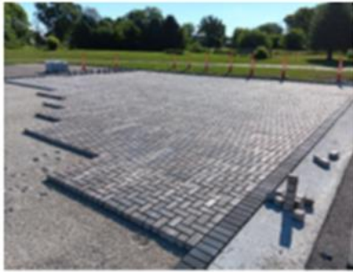
Figure 1: Permeable pavers in place at Fross Park
