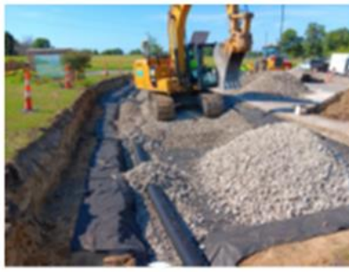
Figure 2: Placing storage aggregate for pavers.
