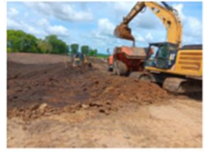
Figure 3: Excavation of the wetland at Mustang Lane.
