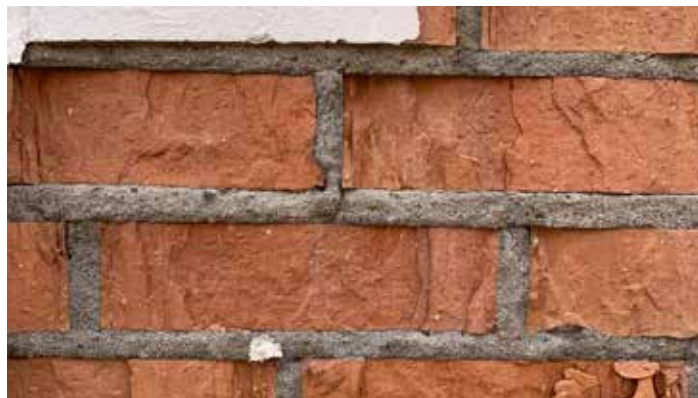
Mortar should be the sacrificial element in masonry; mortar that is too hard can cause damage to the bricks themselves.
