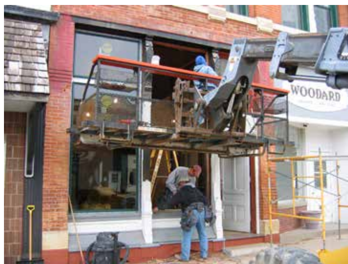
New storefront window frames are constructed between historic cast-iron columns.
