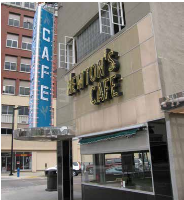
Structural glass panels and thin aluminum frames are character-defining features of this modern-style storefront.
