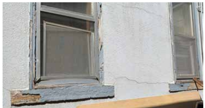
Deferred window maintenance is unsightly and can also affect the thermal performance of a building.
