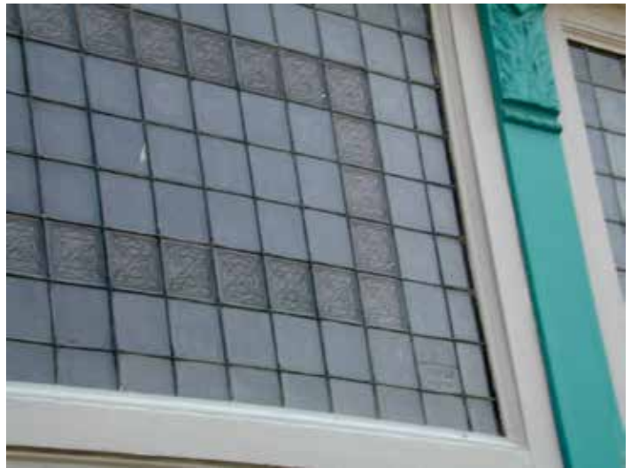
Prism glass was often used in transoms to direct light farther into deep traditional commercial buildings.
