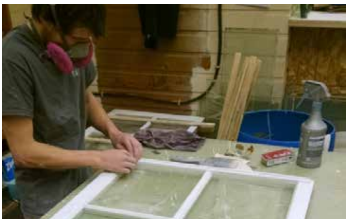
Many wood windows can be rehabilitated by repairing wood sashes, replacing glazing and installing new putty.
