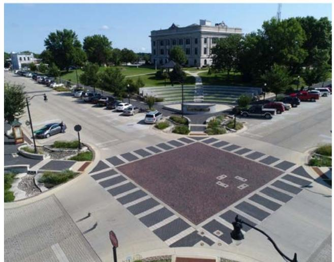
Example of stormwater bumpout intersection
