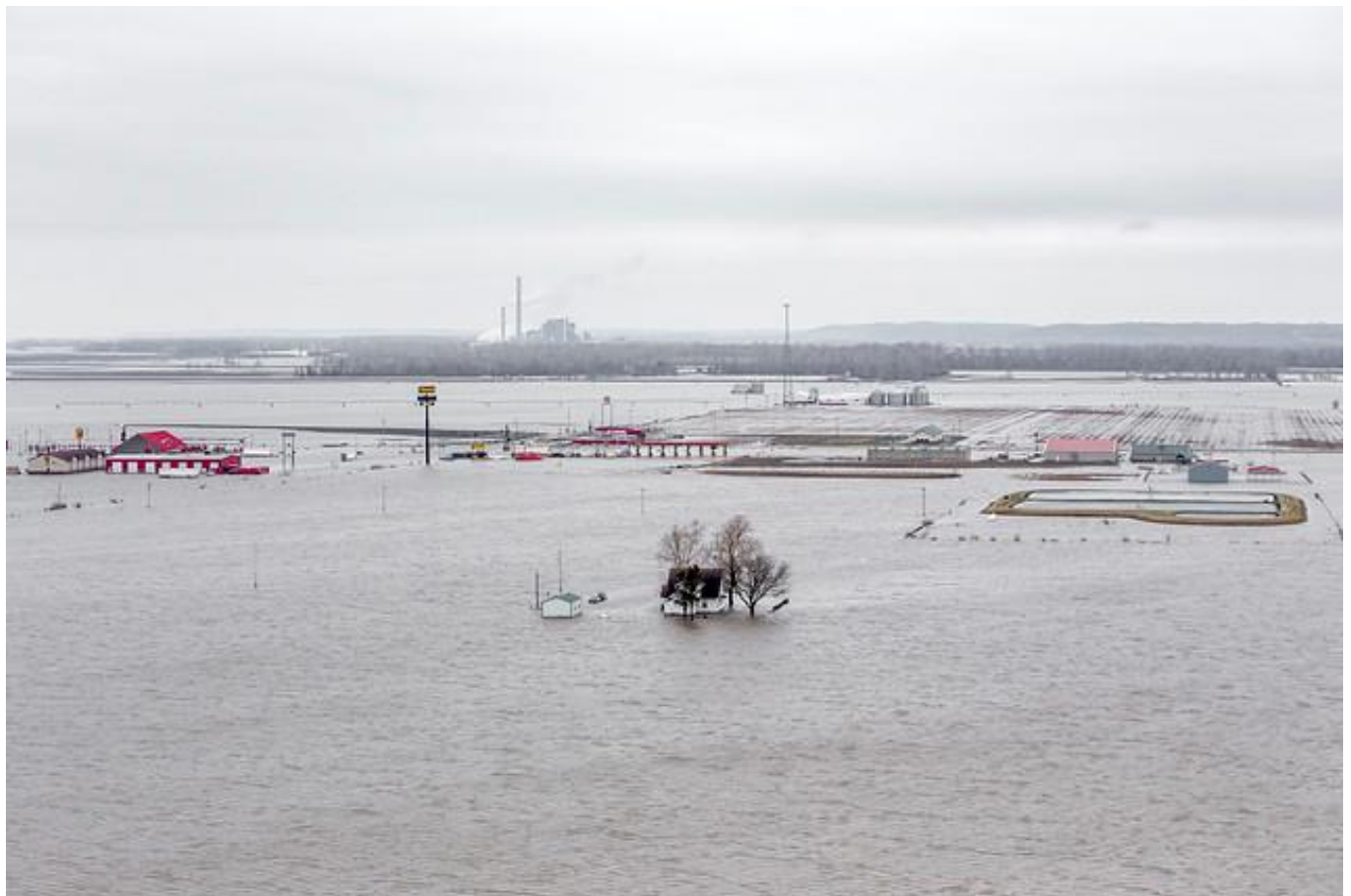
March 28, 2019 – I-29 & US 34 Interchange, Iowa DOT
